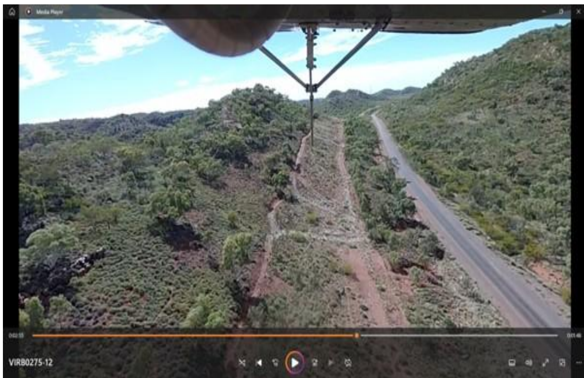
Photo: Rehabilitation work completed to prevent further erosion down slopes (2.55s)
