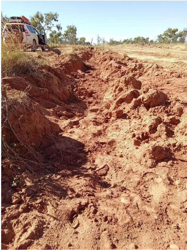
Photo 4-13. Moderate to significant subsidence which has affected a pipeline monitoring pole. KP 5.6
