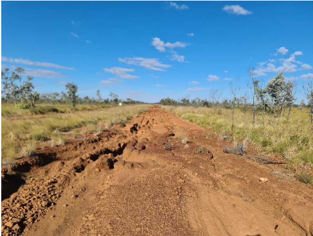
Photo 4-5. Rill erosion scored as the highest severity, Level 1. Erosion had a maximum depth of 1000 mm and the total length of the erosion was approximately 900 m.
