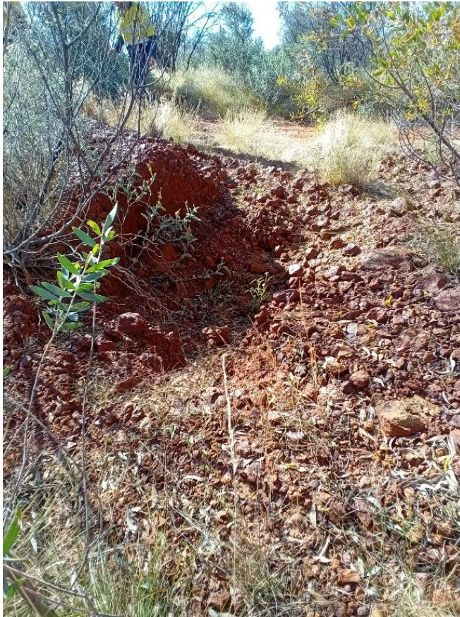
Photo 4-10. Erosion has washed out the middle of a berm at KP 307.5
