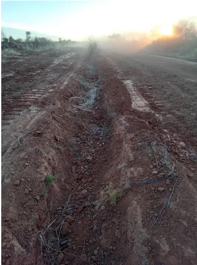
Photo 4-11. Significant subsidence which has not been repaired during grading KP 7
