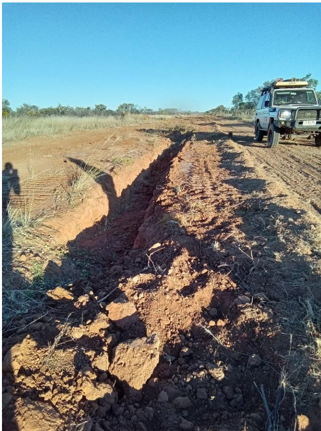
Photo 4-12. Significant subsidence has not been repaired during grading at KP 7.4
