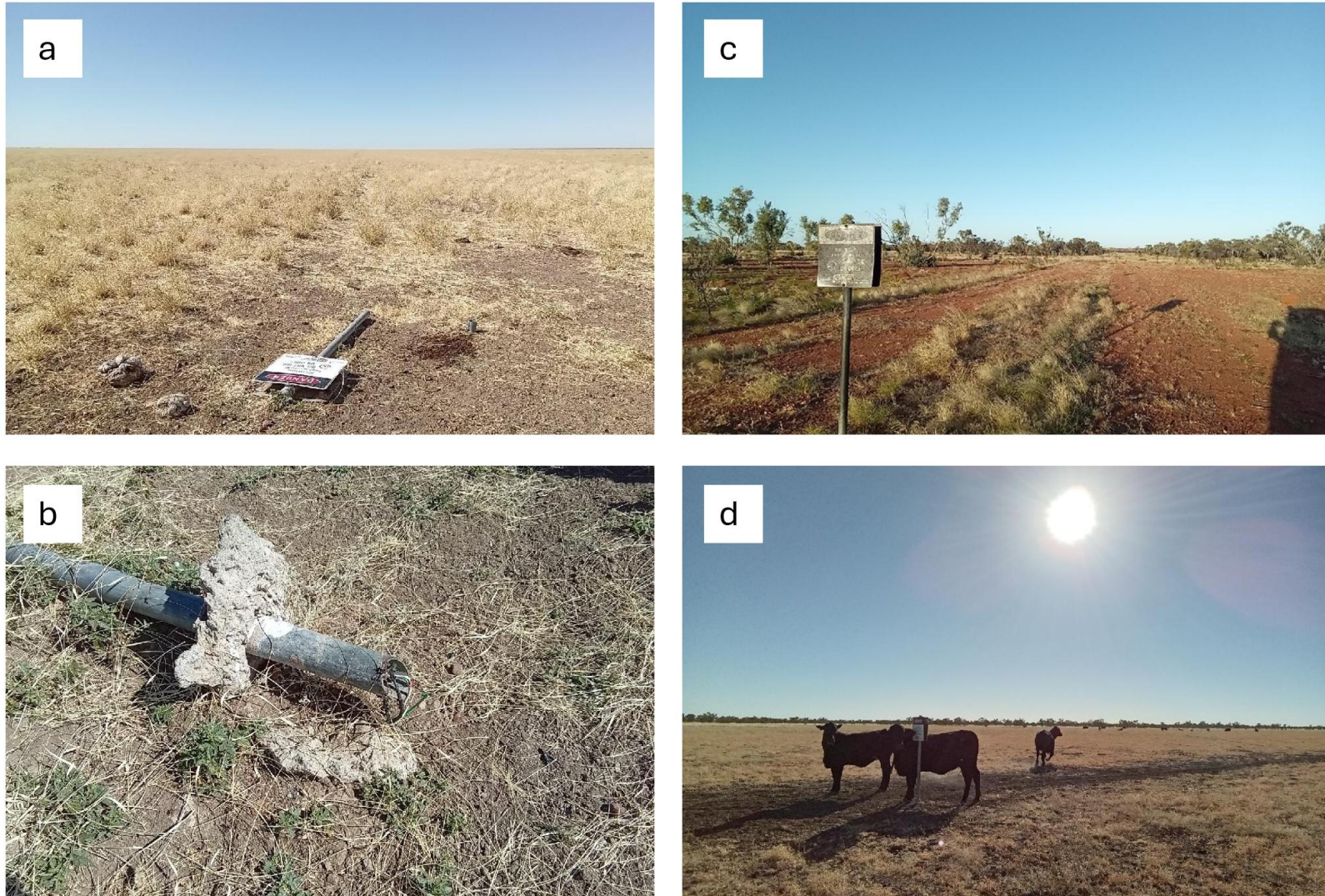
Figure 4-16. Images from the transitional rehabilitation assessment survey: a) fallen sign, b) damaged pole with exposed wires, c) burned sign, d) cattle using sign as scratching post.
