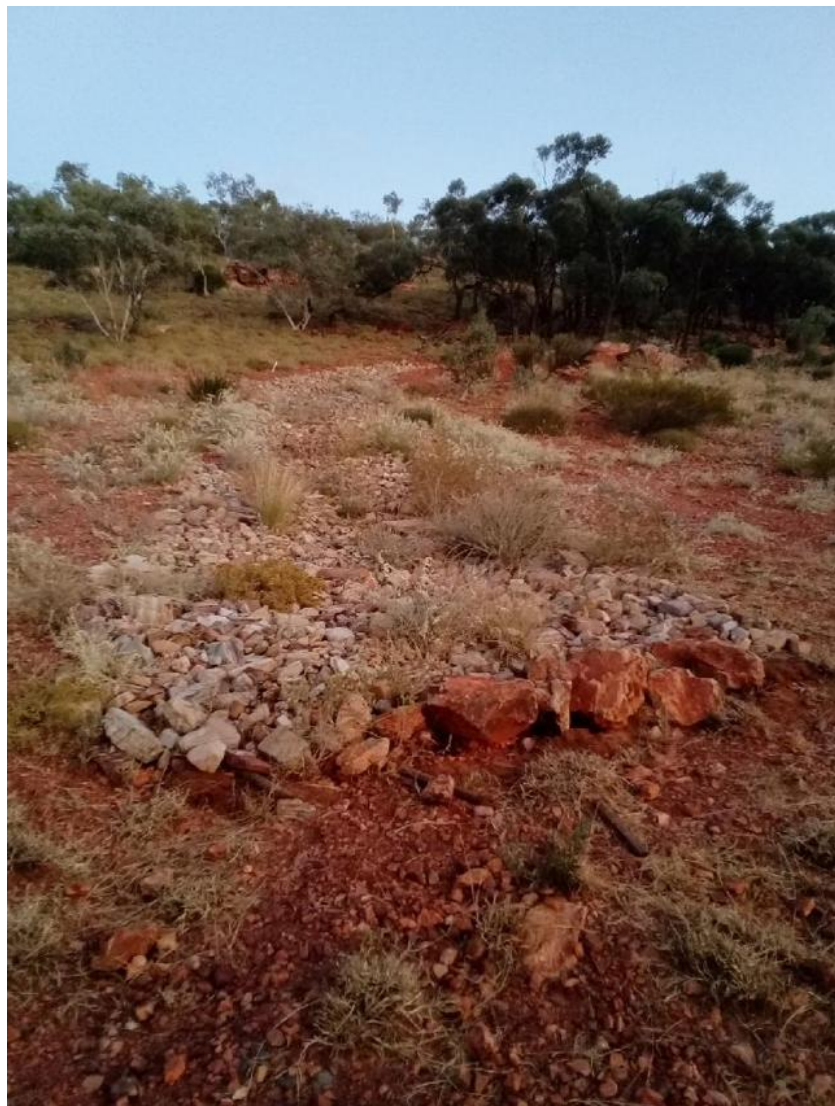
Figure 4-10. Image from the transitional rehabilitation assessment survey: remediated erosion.
