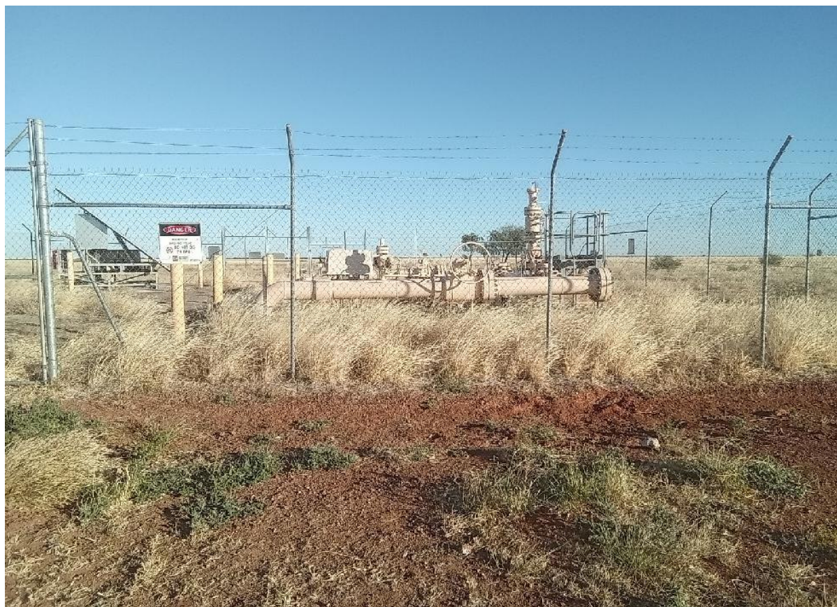
Figure 4-17. Vegetation posing a potential fire risk inside the fencing at Main Line Valve 3.
